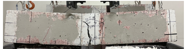
(b) Detail of Failure Mode
