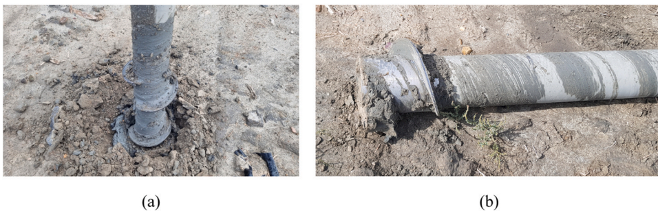
Fig. 8. Results of trial construction of improved FRP screw piles (a) Extraction (b) Failure mode.
