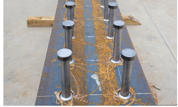
Fig. 2 Bolt Type Shear Connector with Sloped Protrusion
