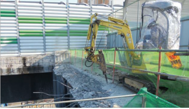
Fig. 1 Concrete Crushing for Replacement of Deck
